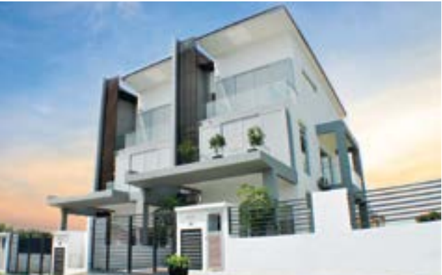
Sunstone Villa (Signature Series 3) - 118 units of the 3-storey villas with a built-up area of 3,040 sq.ft.
