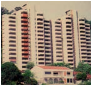
Horizon Towers - Two blocks of 14-storey condominium within the residential area of Tanjung Bungah Park
